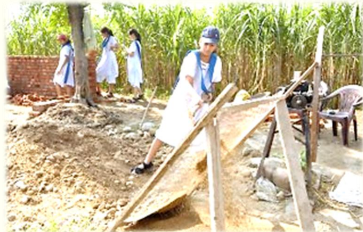
Building Public Toilets in Villages
