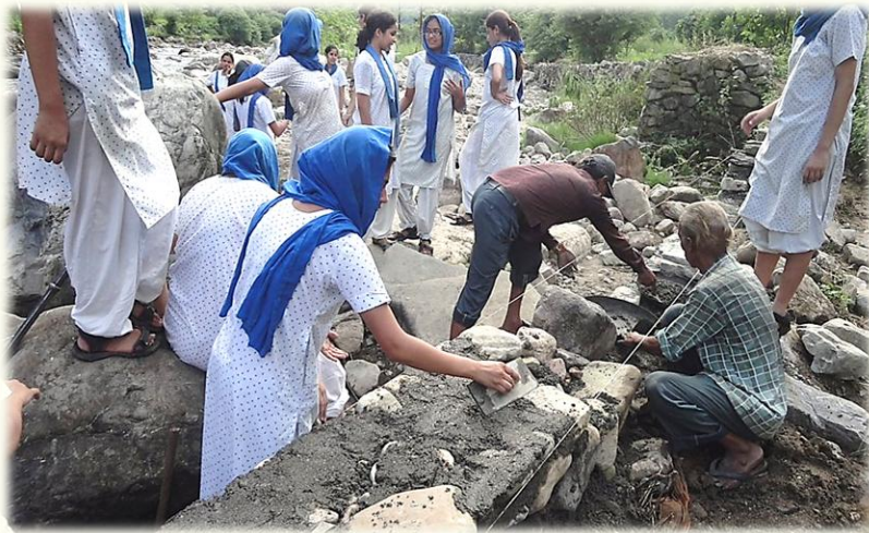
Building a Water Retention Wall
